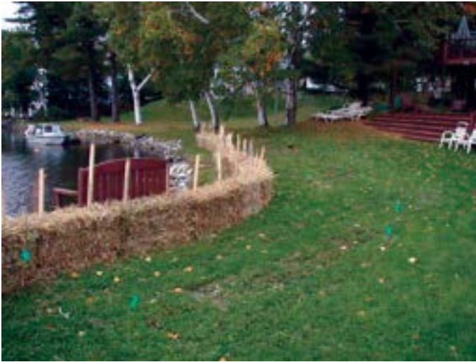
Straw bales protect the water from sediment during a buffer planting.
