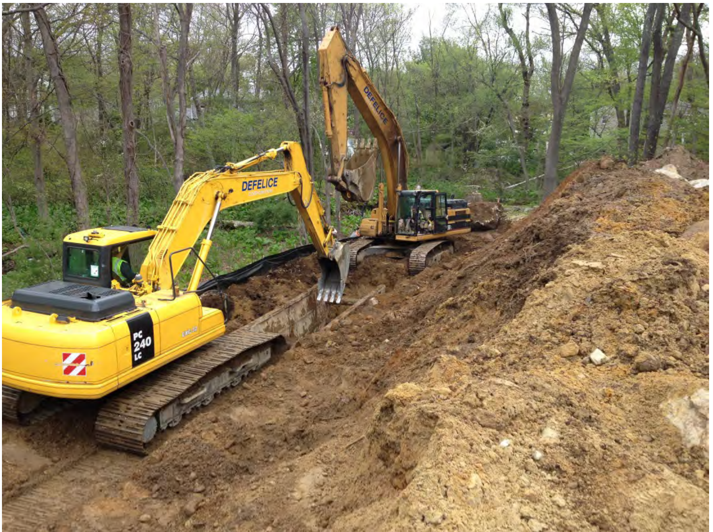
Installing sewer main along the lower back parking lot of the Billerica Elks
